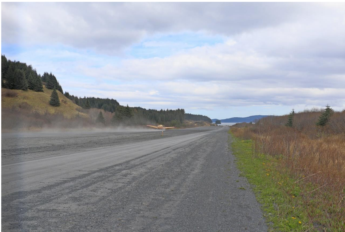
Gravel habitat along runway (N57.88456 x W152.84886)
